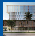
Maroochydore Private Hospital (under construction) Maroochydore City Centre Maroochydore QLD 4558
